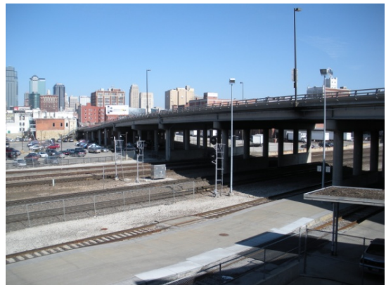
West Face of Prestressed Girder Spans
