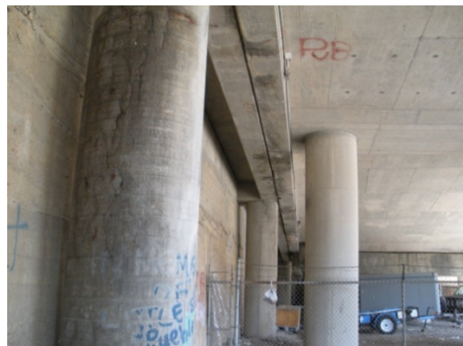
East Column of Bent 2N
