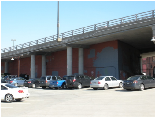
West Face of Voided Slab Spans
