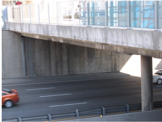
West Face of Bridge
