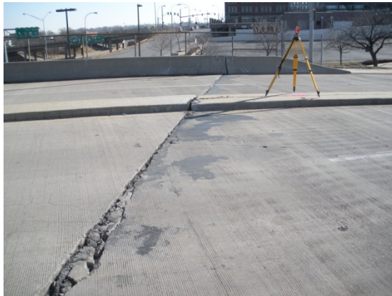
Approach Slab Joint at South End Bent
