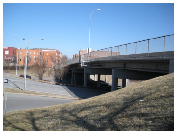
West Face of Bridge
