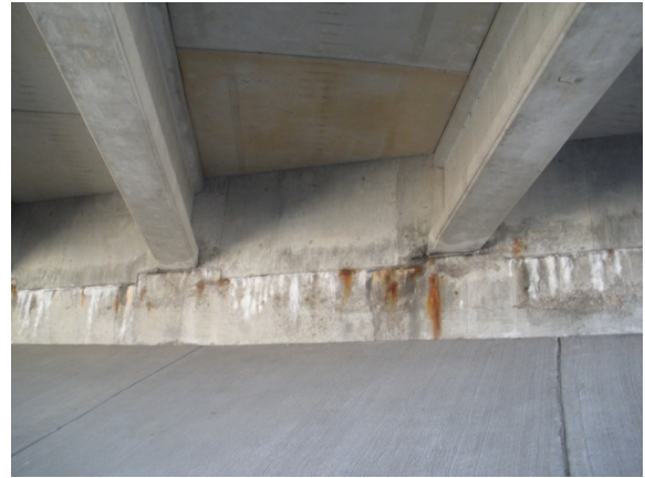
South End Bent
